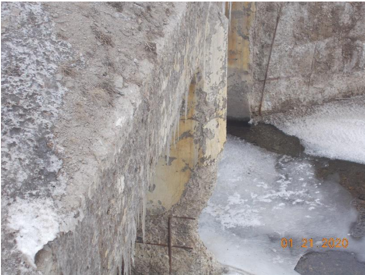
Paint sample G-12-C-LP01. The tan paint on the concrete is considered lead containing paint.
