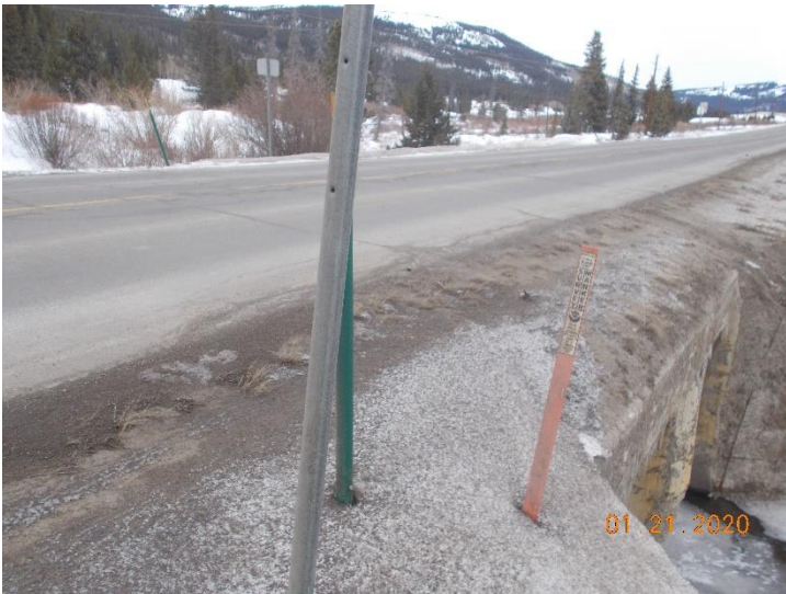
View of bridge G-12-C looking north.
